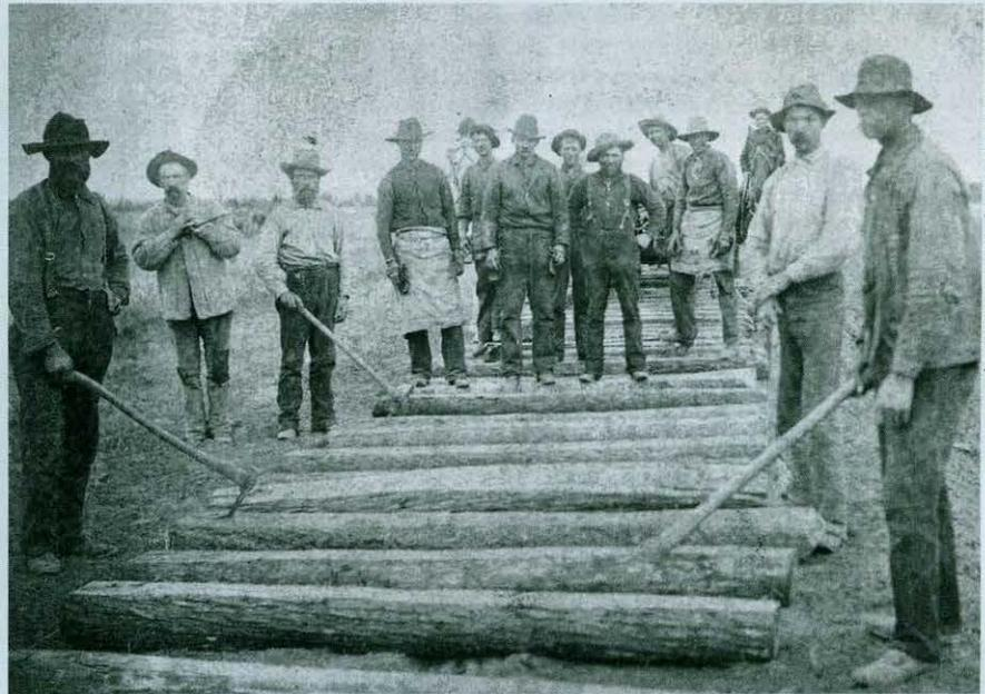
Above, tie crews of the Montana Central Railroad position ties using picaroons. The Central line extended the St. Paul, Minneapolis & Manitoba line to Helena and Butte after its completion to Great Falls in fall 1887.
